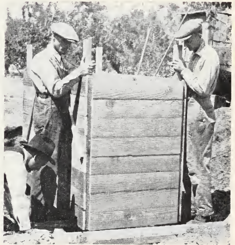
Fig. 11—The completed form being lowered into the hole.
